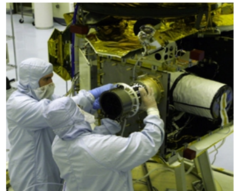
Figure 14-3: Picture of SWAP being mounted to the spacecraft.
